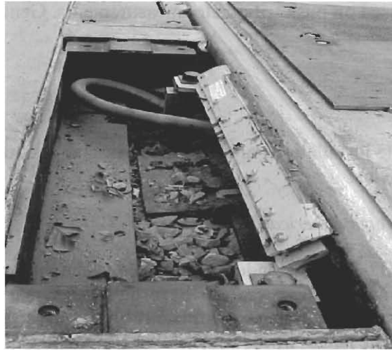
Fig. 7. Top of rail bars installed on imbedded track.
