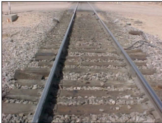
Figure 5: Cribs 1 & 2 in Tangent Section (Bungalow 1)
